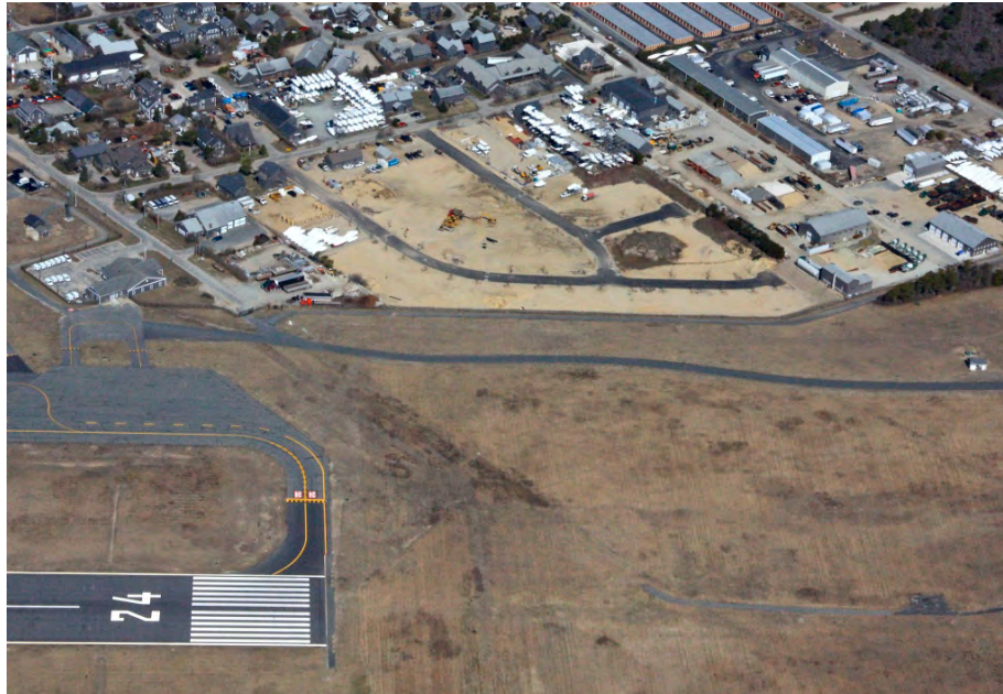
Figure 2-45 – Development in Coffin Pit Abutting Runway 24 (view looking north)
