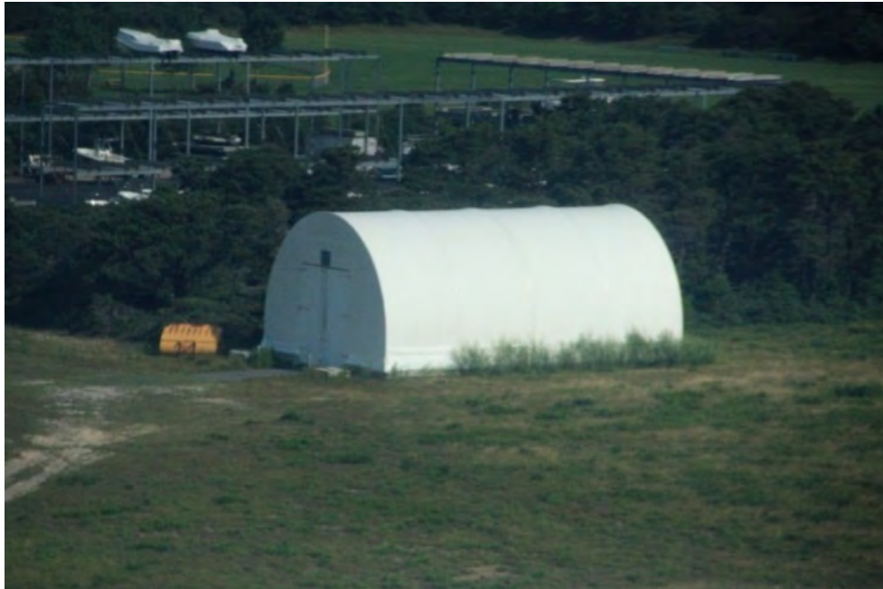
Figure 2-26 – SRE Temporary Tent Storage Structure
