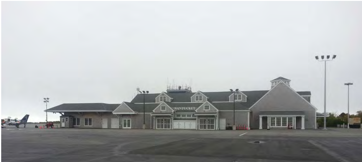
Figure 2-30 – View of the Terminal Expansion from the North Apron
