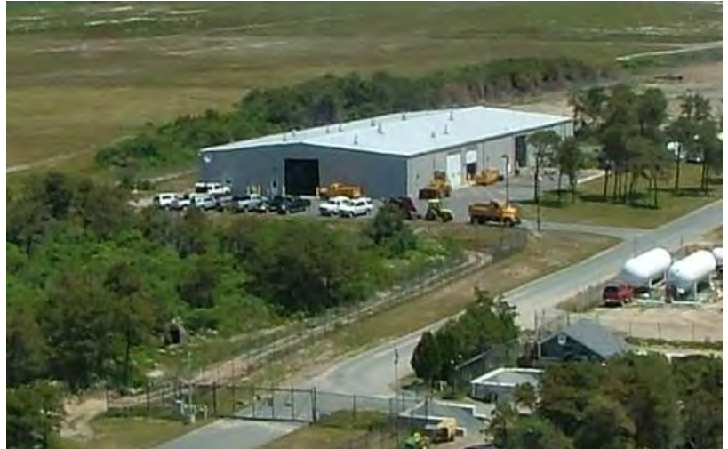
Figure 2-24 – SRE Maintenance Garage
