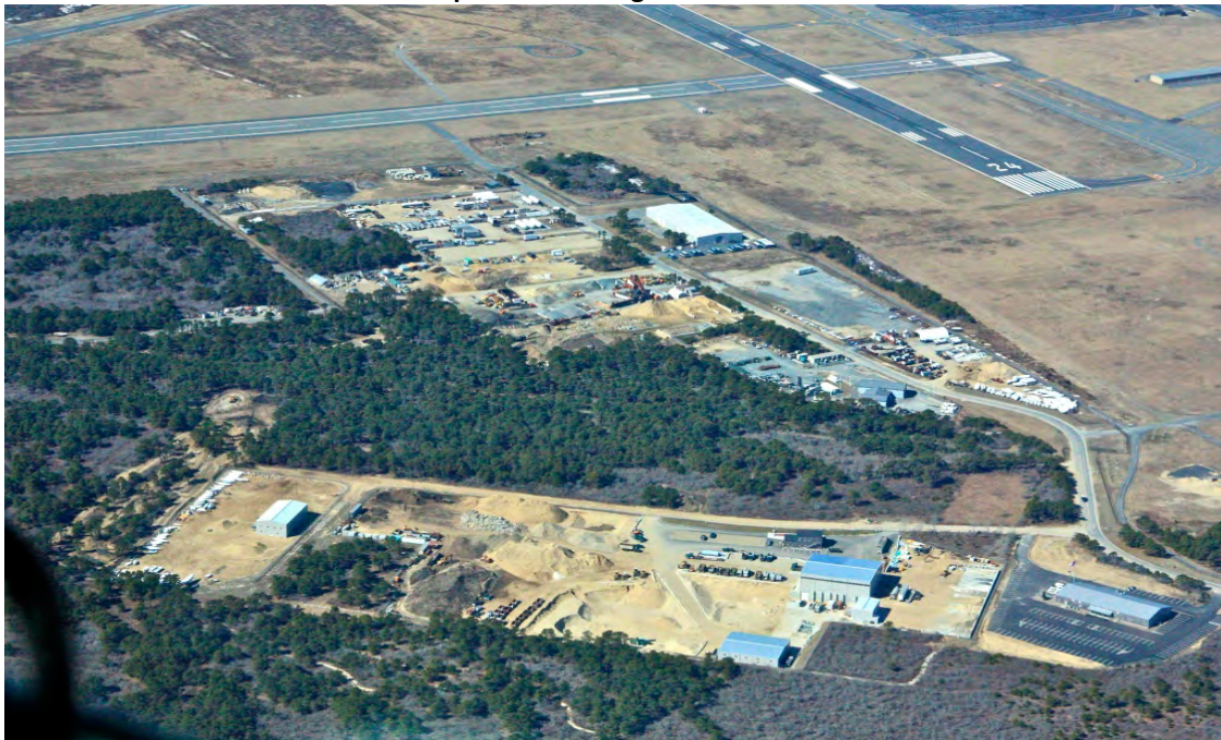
Figure 2-44 – Commercial Industrial Development Abutting the Bunker Area
