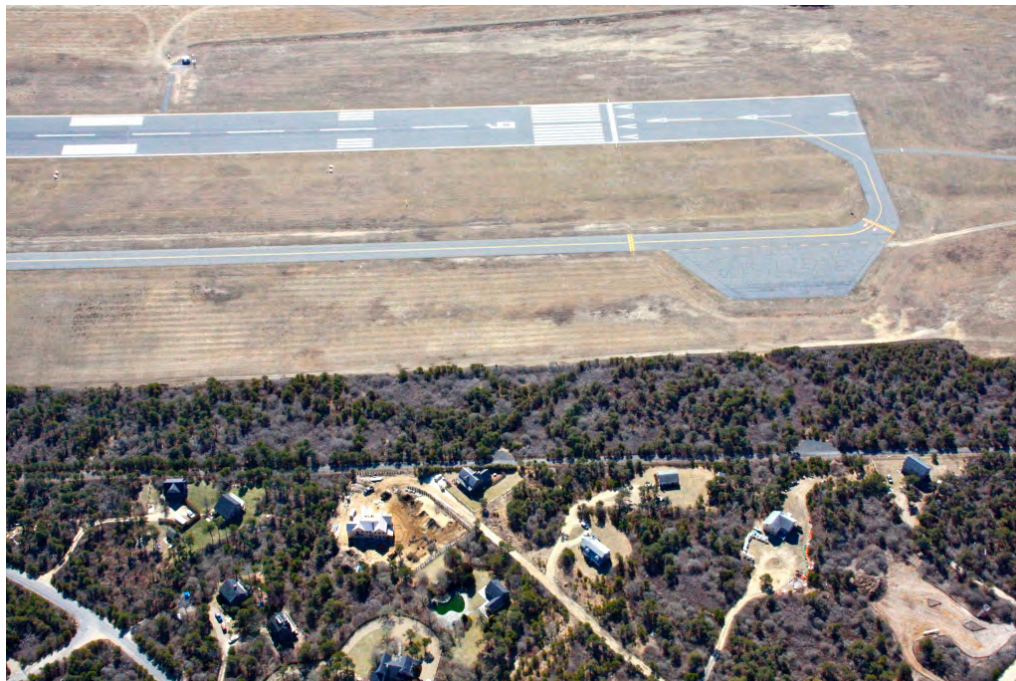
Figure 2-46 – Residential Development Abutting Runway 6 (view looking south)
