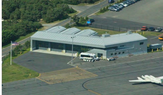
Figure 2-28 – ACK ARFF Building and ARFF Truck
